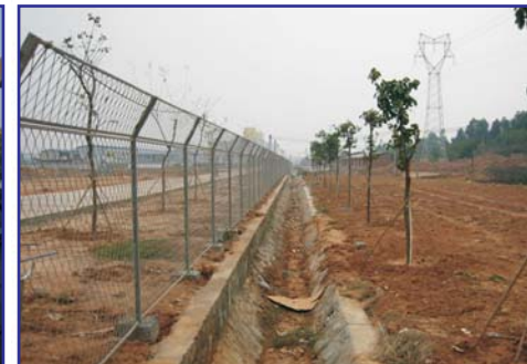
Factory compound surrounded by a fence in Guangzhou
